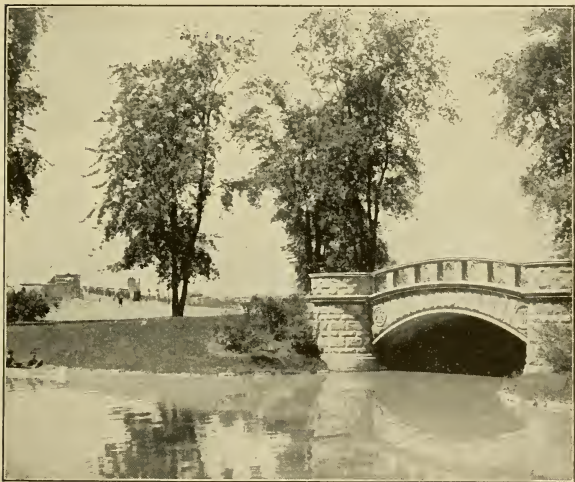
Entrance to Belle Isle from the Bridge.
